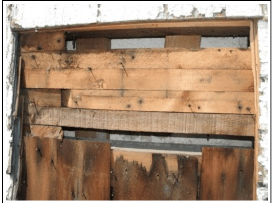
Photo. 1: An image extracted from a 2014 investigation report by Scheinman and Silburn which illustrates varying conditions within an area where shingles were removed to reveal underlying woodwork.
