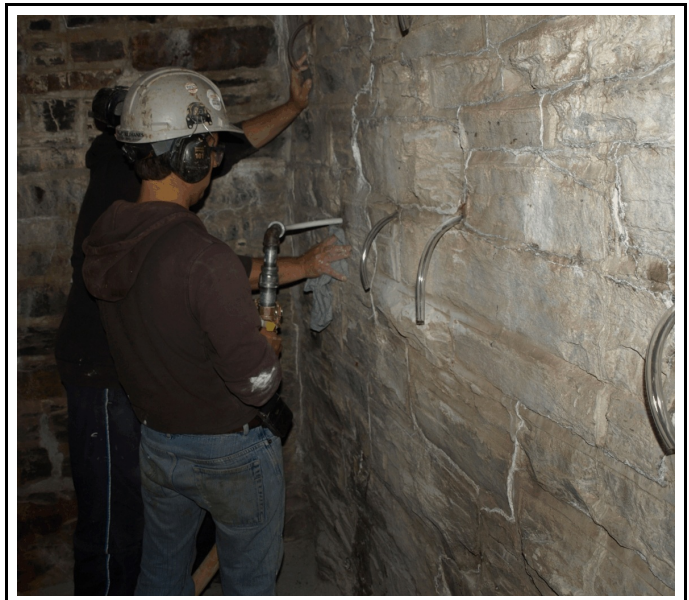
Photo. 13: Using low pressure to inject the cellular foamed cement grout into a traditional mass masonry wall. (Dingle Tower, Halifax)
