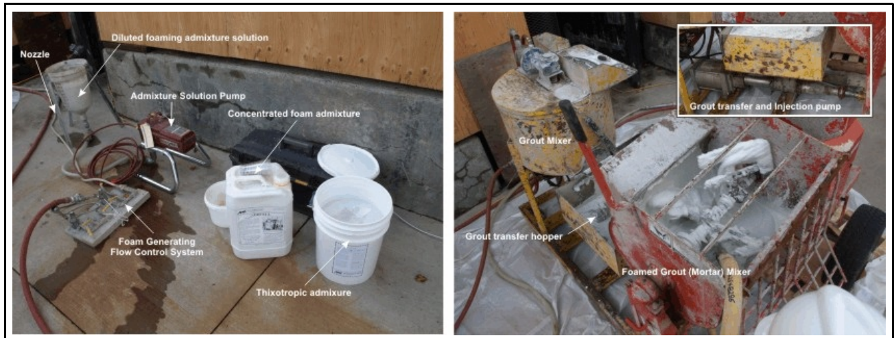
Photo 11: (Left) Equipment and materials for generating foam. Photo 12: (Right) Equipment set up for producing foamed grout.
