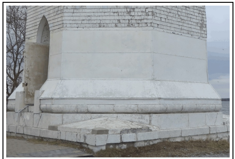
Photo. 3: Illustration of the metal cladding at the base of the tower above the stone foundations.
