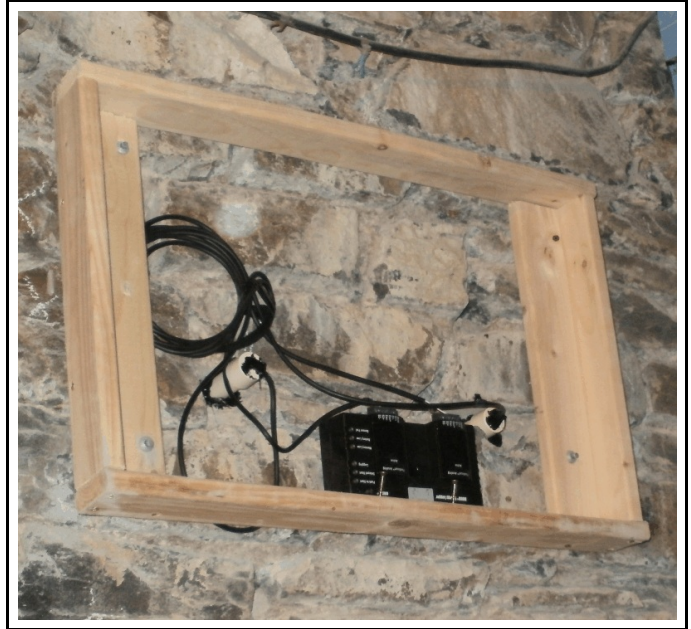
Photo. 14: Example of installed sensors set to monitor moisture conditions within a tower's masonry assembly.
