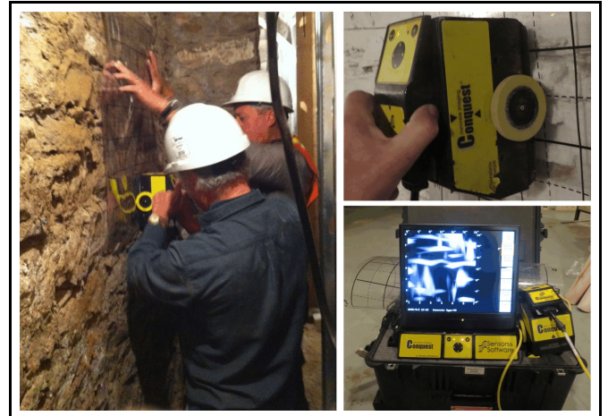
Photo. 4 (left): Scanning a location using Ground Penetrating Radar. Photo. 5 (upper right) The scanning head moved over a temporary grid. Photo 6. (Lower right): A typical scan of a grid slice visually interpreted by the computer.
