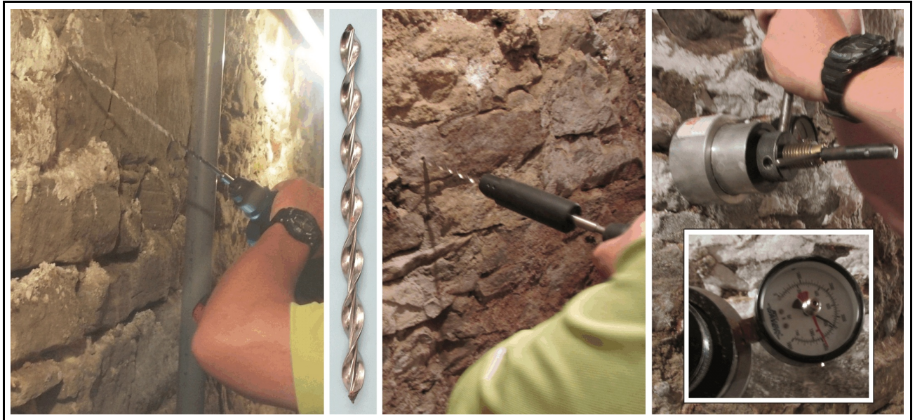
Photo.7 : (Left) Installing a stainless steel helical masonry tie. Photo. 8: (Second from left) An illustration of a stainless steel helical masonry tie. Photo. 9 : (Centre) Installation of a tie within a pilot hole. Photo. 10: (Right with inset image.) Testing an installed tie using a pull-off testing device to apply an axial load.
